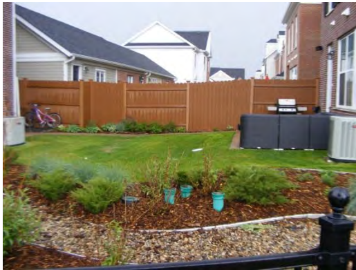
Infiltration trench
