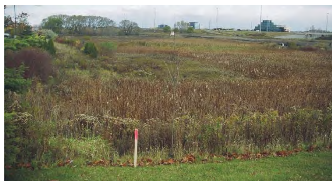
Dry stormwater pond
