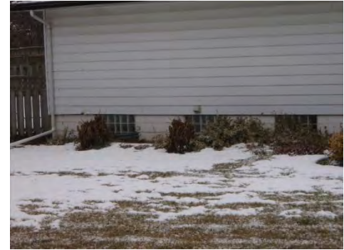
Sealed Glass Block Basement Windows to Provide Flood Proofing
