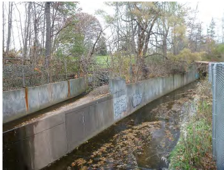
Concrete Lined Diversion Channel
