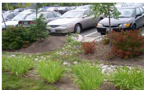
Bioretention cell in a commercial parking area
