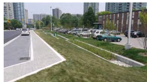
PICP lay-by and sidewalk, Mississauga, ON
