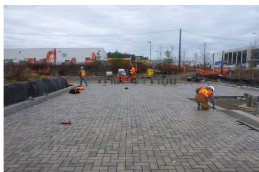
PICP parking lot
