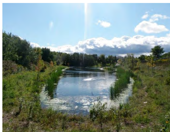
Wet stormwater quality pond
