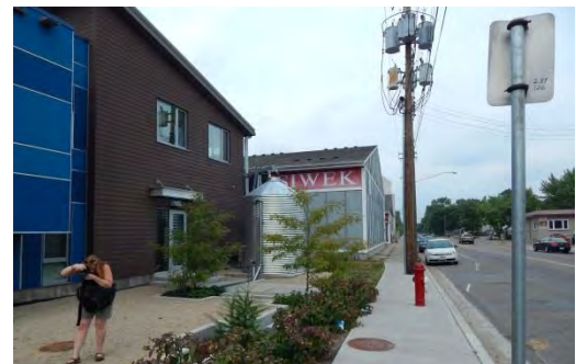
Rainwater Harvesting (Employment Building) St. Paul, Minnesota
