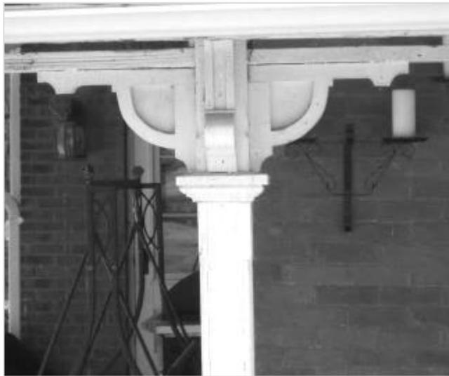
*Apply traditional joining details. The use of dovetail, tenon and mortise, dowels, and splines is more preferred over metal fasteners during repair*
