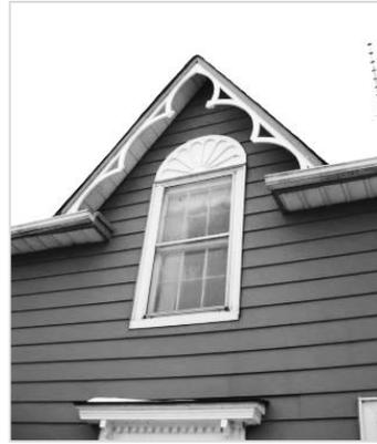
*Wooden millwork is typical of 19th Century Ontario architecture. Timber is a capable material to hold glass for operable windows, and with proper maintenance, can endure harsh weather conditions*
