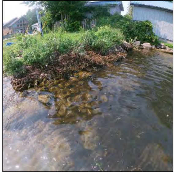
Image 2: Existing impacts and gabion wall.
