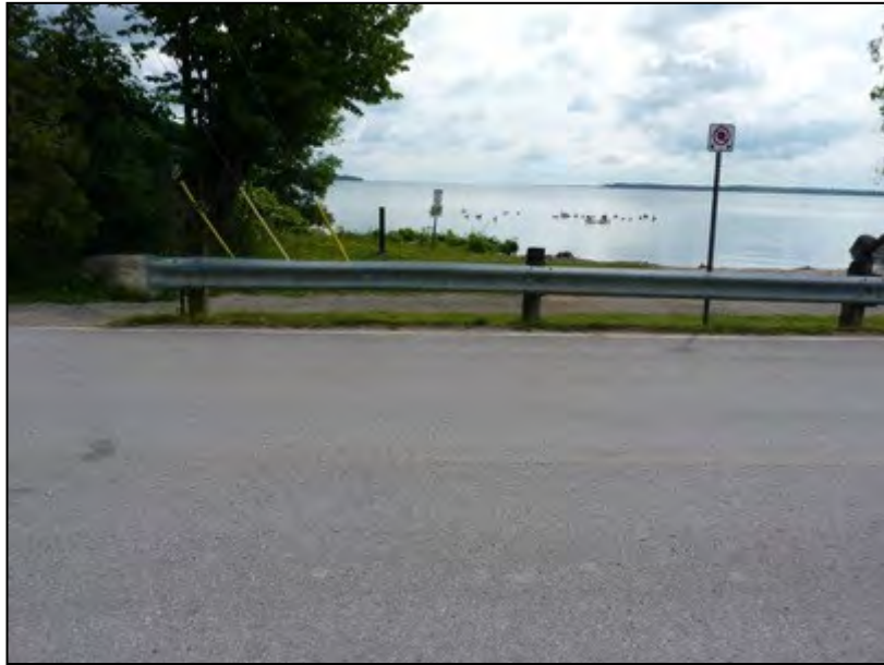
Image 1: Shows disturbed areas at Roberts Road Outlet.
