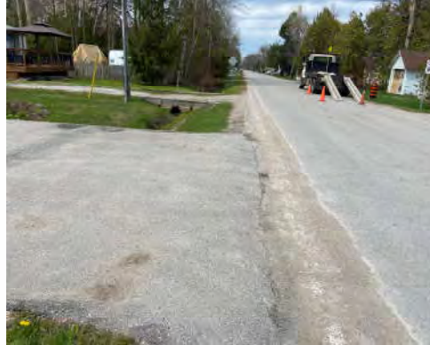
Existing Crystal Beach Rd Ditch Looking North from South End
