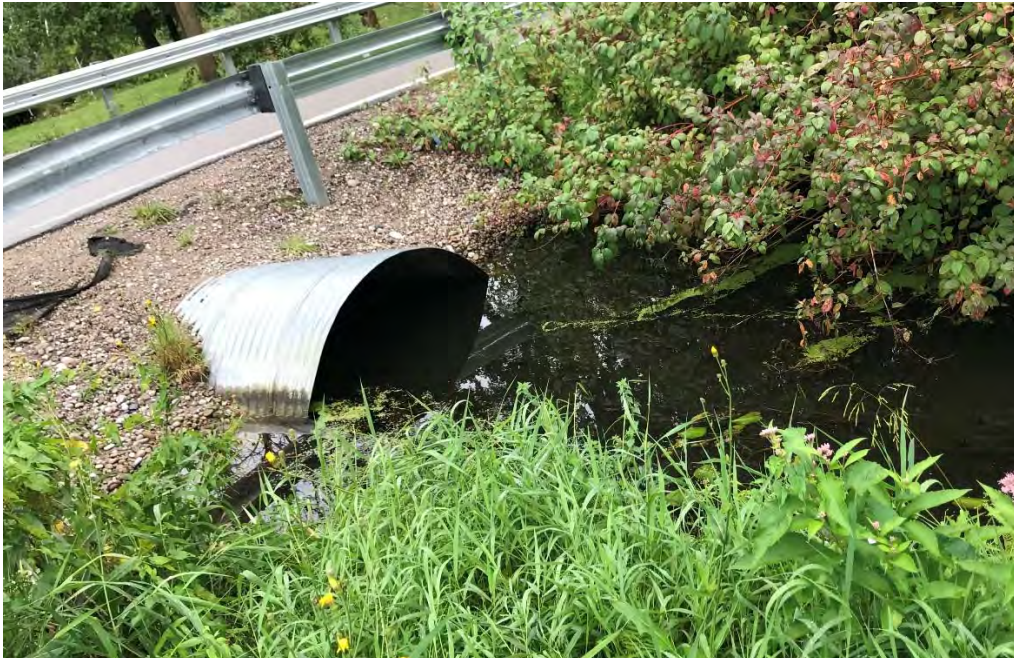
Photograph 12: Goodfellow Avenue 2100 mm Dia. Culvert Crossing Inlet
