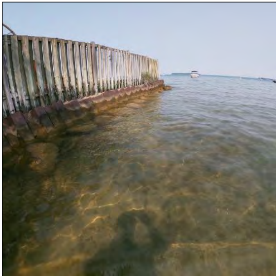
Image 3: Steel piling wall forming the northern limit of the Study Area.
