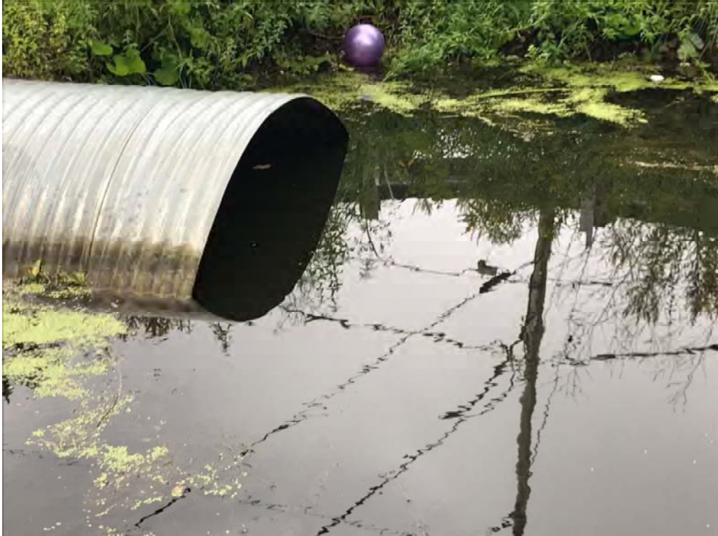
Photograph 13: Goodfellow Avenue 2100 mm Dia. Culvert Crossing Outlet
