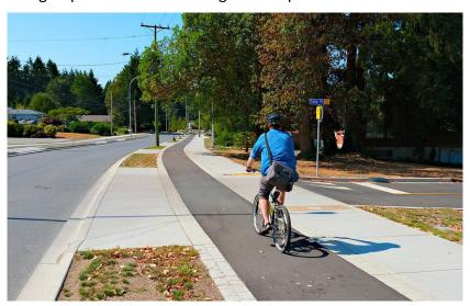
Figure 37: Example of a continuous sidewalk and cycle track implemented on Metral Drive in Nanaimo, BC (Source: Roy Symons on Flickr)
