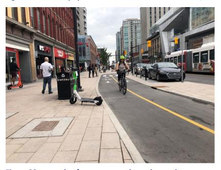
Figure 28: example of a two-way cycle track on a downtown street
