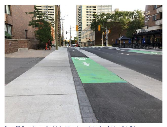
Figure 36: Example use of a strip to delineate a cycle track and sidewalk in Ottawa
