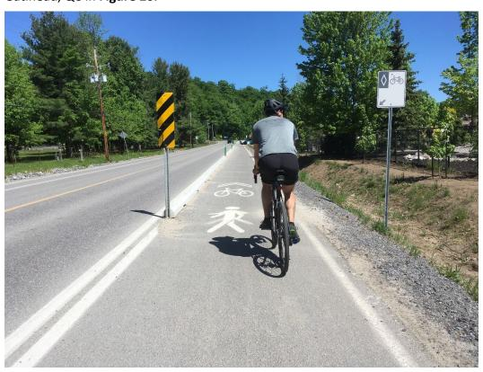
Figure 26: Example of rural paved shoulders separated from vehicle lanes by pinned curbs and bollards in Gatineau, QC
