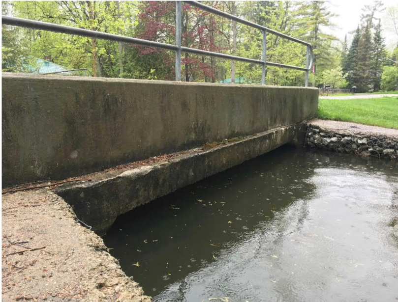
Figure 3-6: Existing Cross Street Culvert Structure
