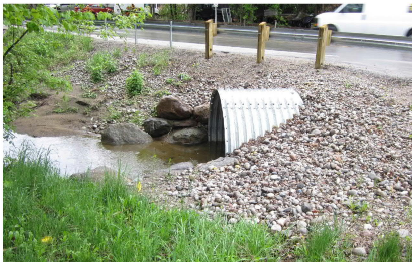
Figure 5-1: Existing CSP Culvert at St. Johns Road and 7 th Line
