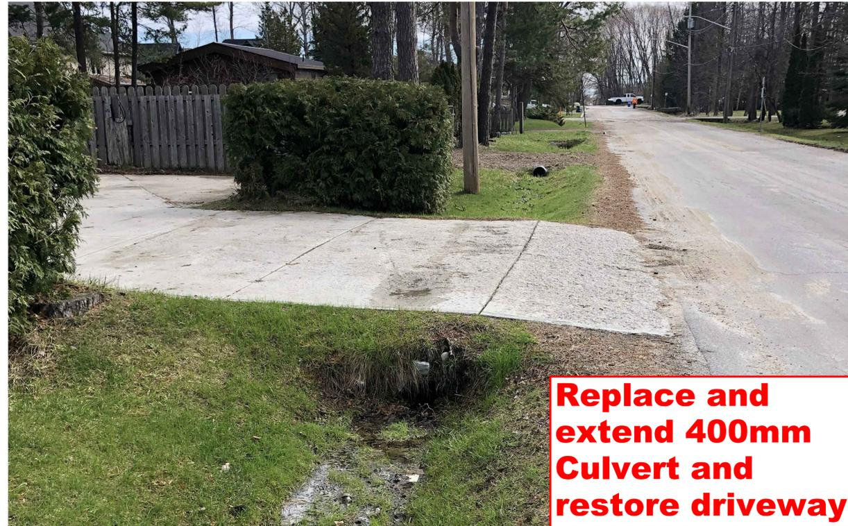
**Replace and extend 400mm Culvert and restore driveway**
