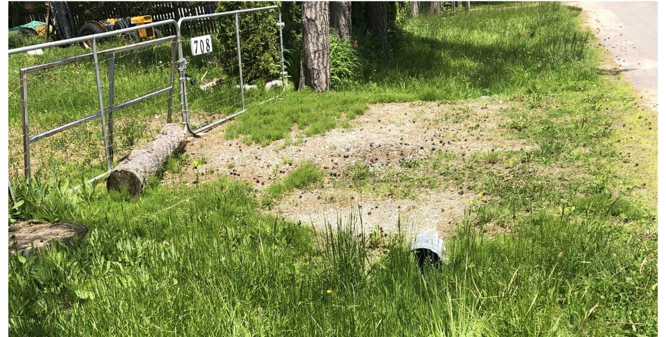
**Replace, extend & upgrade with 500mm Culvert and restore driveway**
