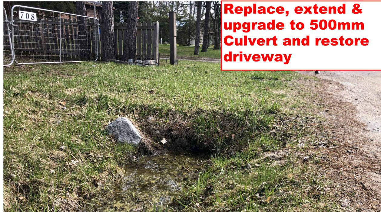
**Replace, extend & upgrade to 500mm Culvert and restore driveway**
