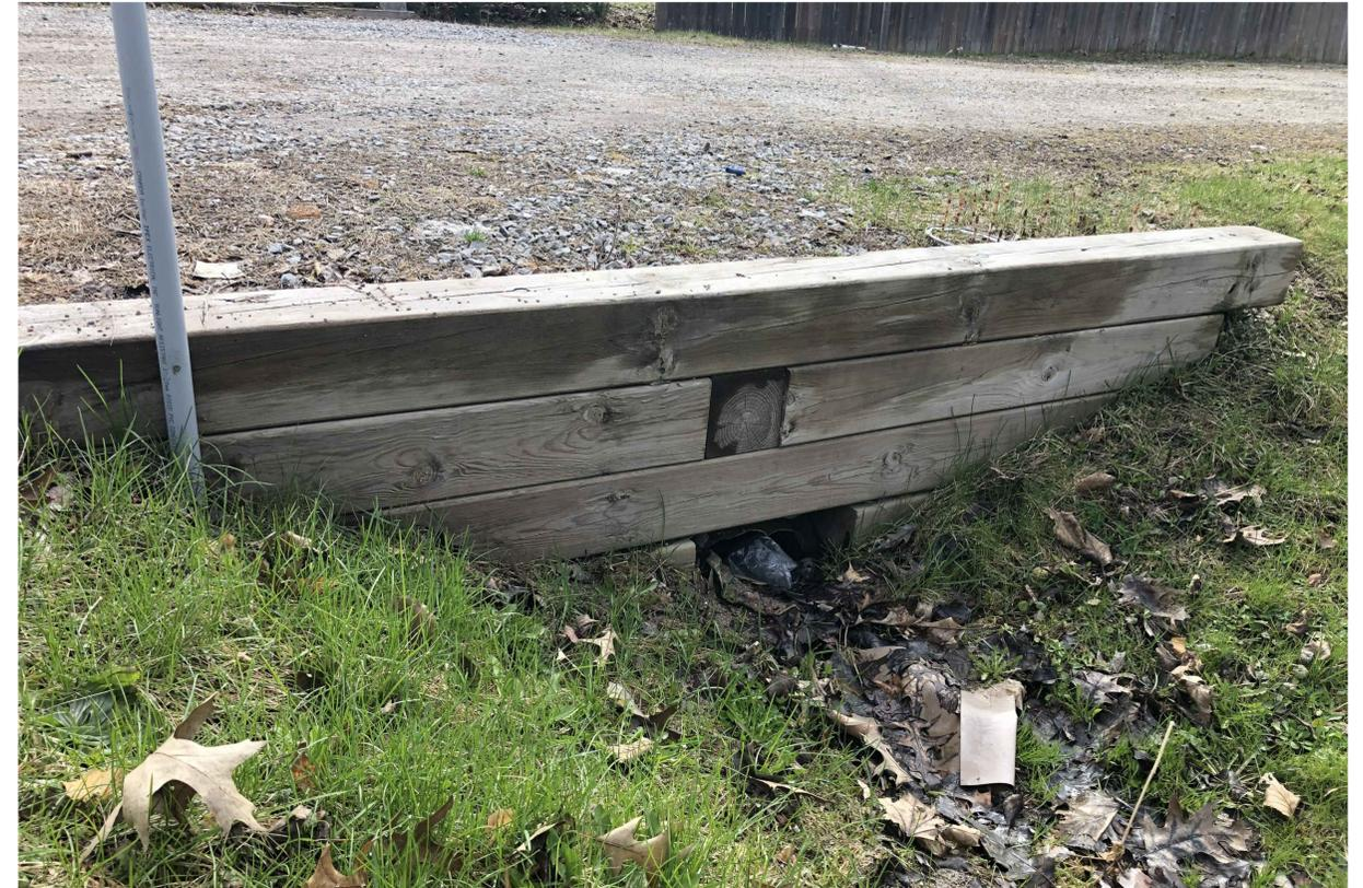
**Replace, extend & upgrade to 400mm Culvert, remove headwall and restore driveway**
