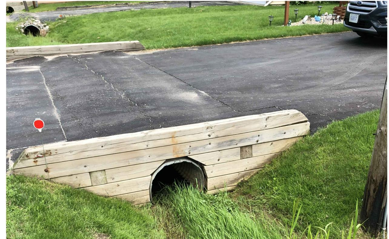
**Replace and extend 600mm Culvert, remove headwall and restore driveway**
