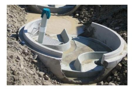
Oil and Grit Separators (OGS) are underground devices that are attached to storm sewer pipes. They remove sediment, screen debris, and separate floatables like oil and grease.
