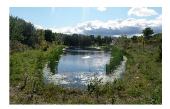
Stormwater management ponds collect and store stormwater to reduce flooding and erosion by limiting the release of water to nearby creeks and rivers.
