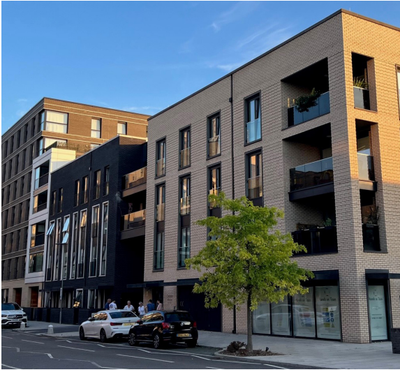
Figure 40: Continuous streetwall of mid-rise buildings
