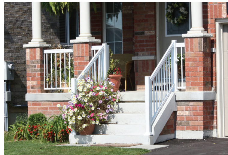
Typical stair detail, where more than 4 risers are required
