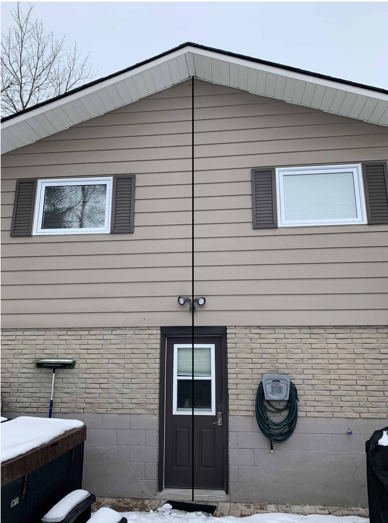
HEIGHT OF RESIDENCE - GRADE TO UNDERSIDE OF SOFFIT AT REAR 6.22 m (20'-4 3/4")
