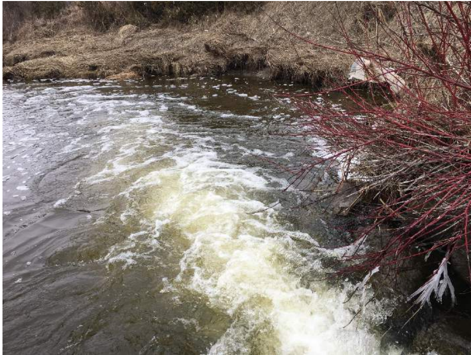
Photo 11: Looking west, the outlet of the single CSP beneath Highway 400 (April, 2018).
