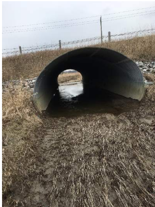
Photo 12: Looking east, the inlet to the southern CSP culvert beneath Reive Boulevard (April, 2018).
