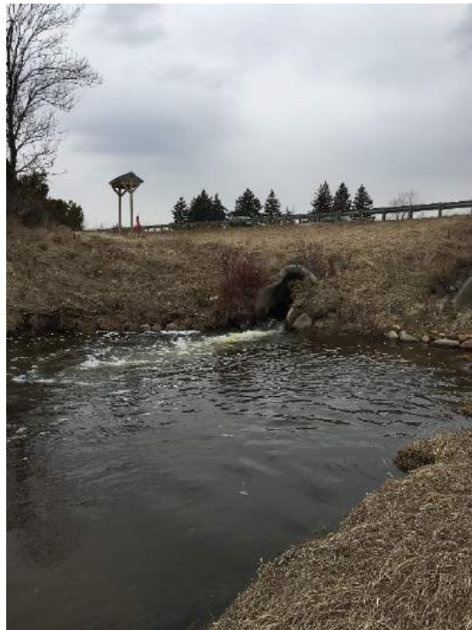
Photo 8: Looking east, the outlet of the single CSP beneath Highway 400 (April 2018).
