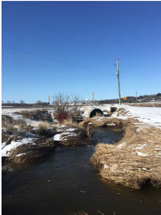
Photo 28: Looking south, the Inlet of the 4 th Line CSP culverts (April, 2018).
