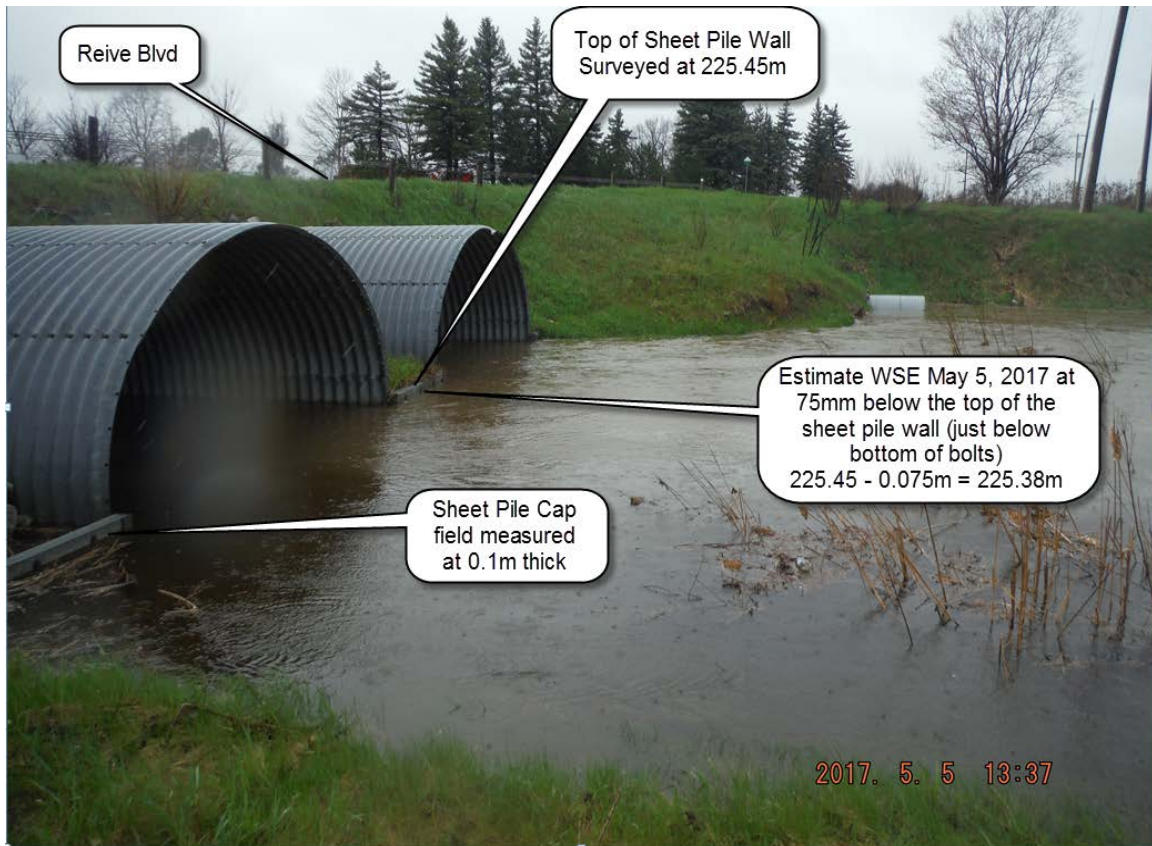
Figure 13 May 5, 2017 Rainfall Event – Upstream Limits of Reive Boulevard
