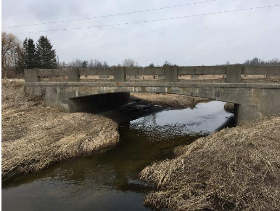
Photo 17: Looking north, the Drain flowing through the 2 nd Line Crossing. (April, 2018).
