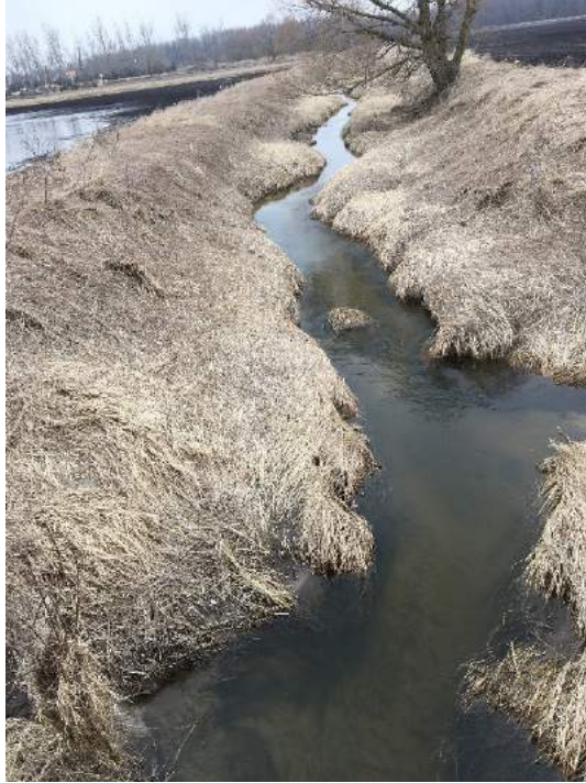
Photo 23: Looking north, the Drain flowing upstream of 3 rd Line (April, 2018).
