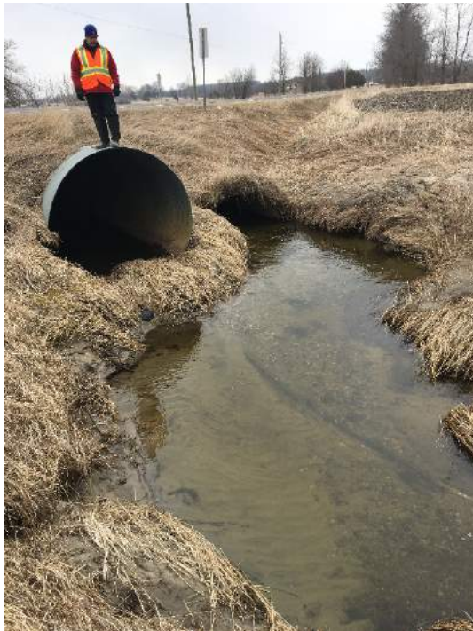
Photo 26: Looking north, the outlets of the culverts beneath 4 th Line (April, 2018).
