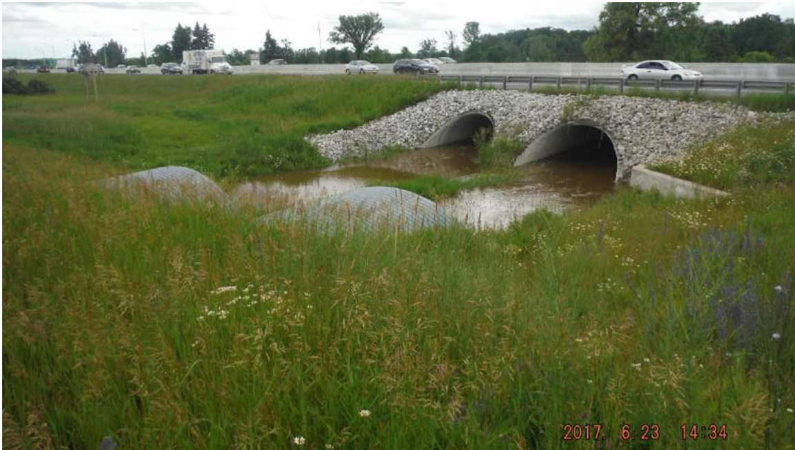
Figure 4 Existing Highway 400 Culvert Crossings – Upstream View
