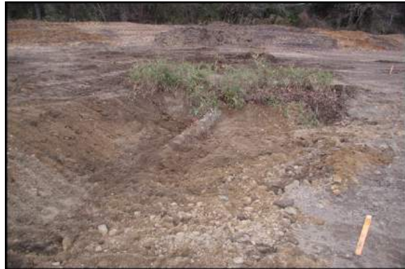
Photo 32. Sod mat placed to form stream bank. Source: Buck Engineering
