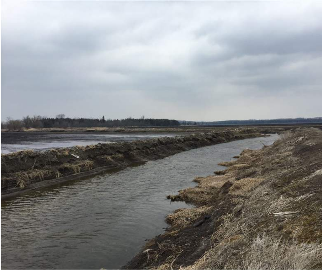
Figure 7 Existing Drain Configuration STA 2+300 to STA 6+120
