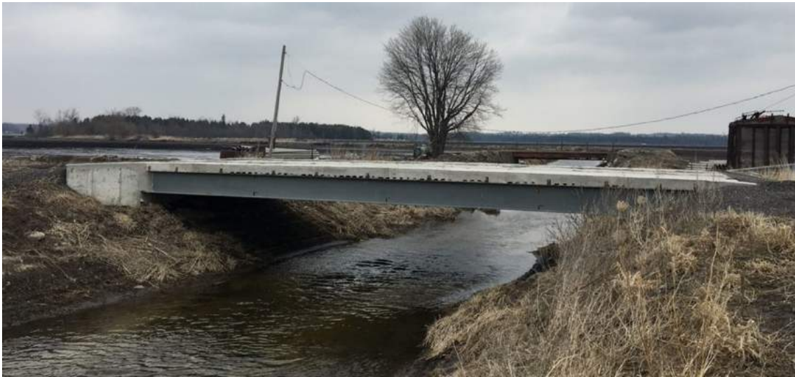
Figure 20 Drain Crossing at STA 4+359
