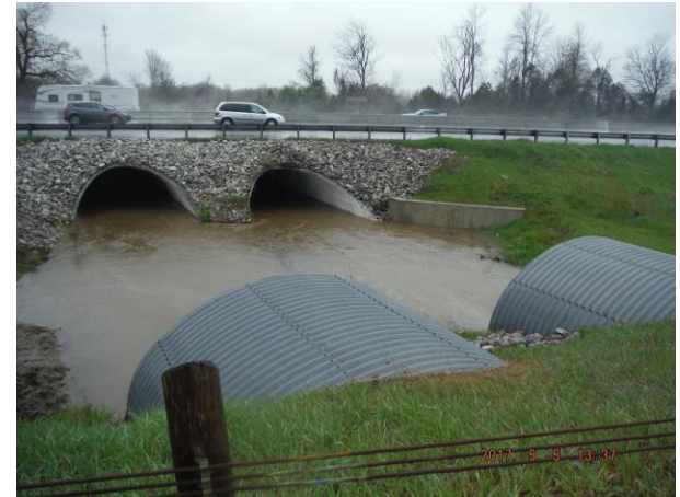
Looking Downstream from Reive Blvd.
