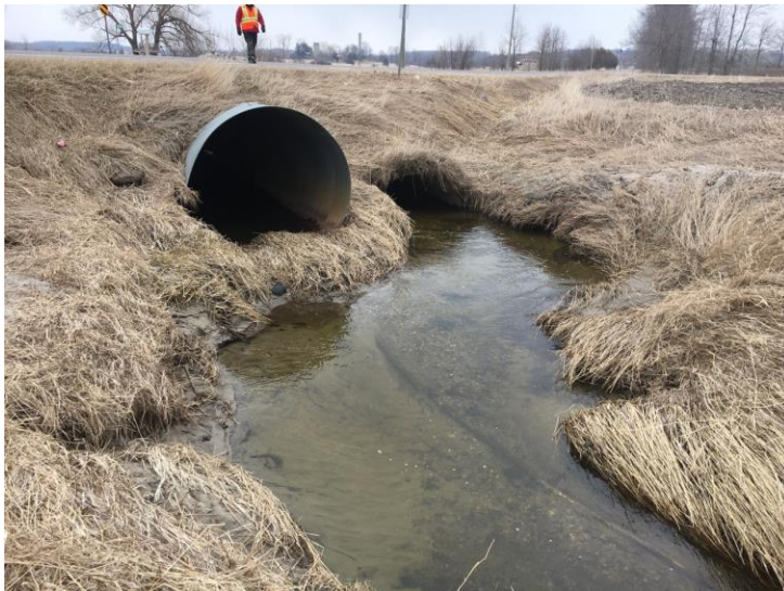
4th Line Crossing – Main Drain
