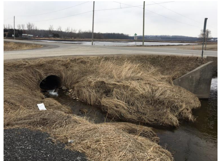
3rd Line Crossing – 10 Sideroad Branch Drain
