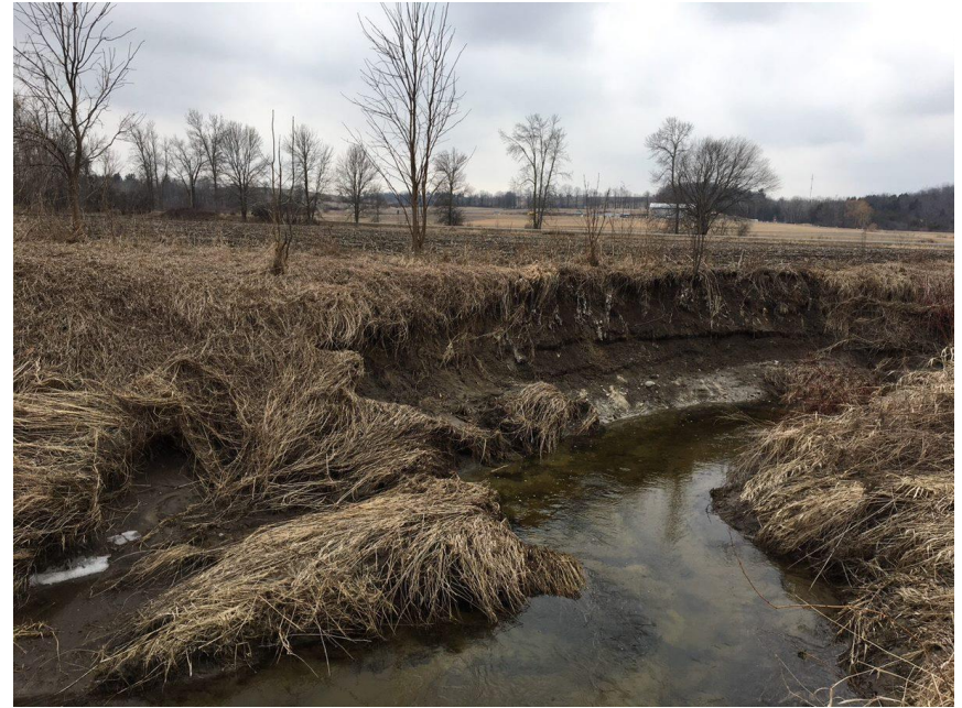
Lot 6, Concession 1 - Looking Upstream
