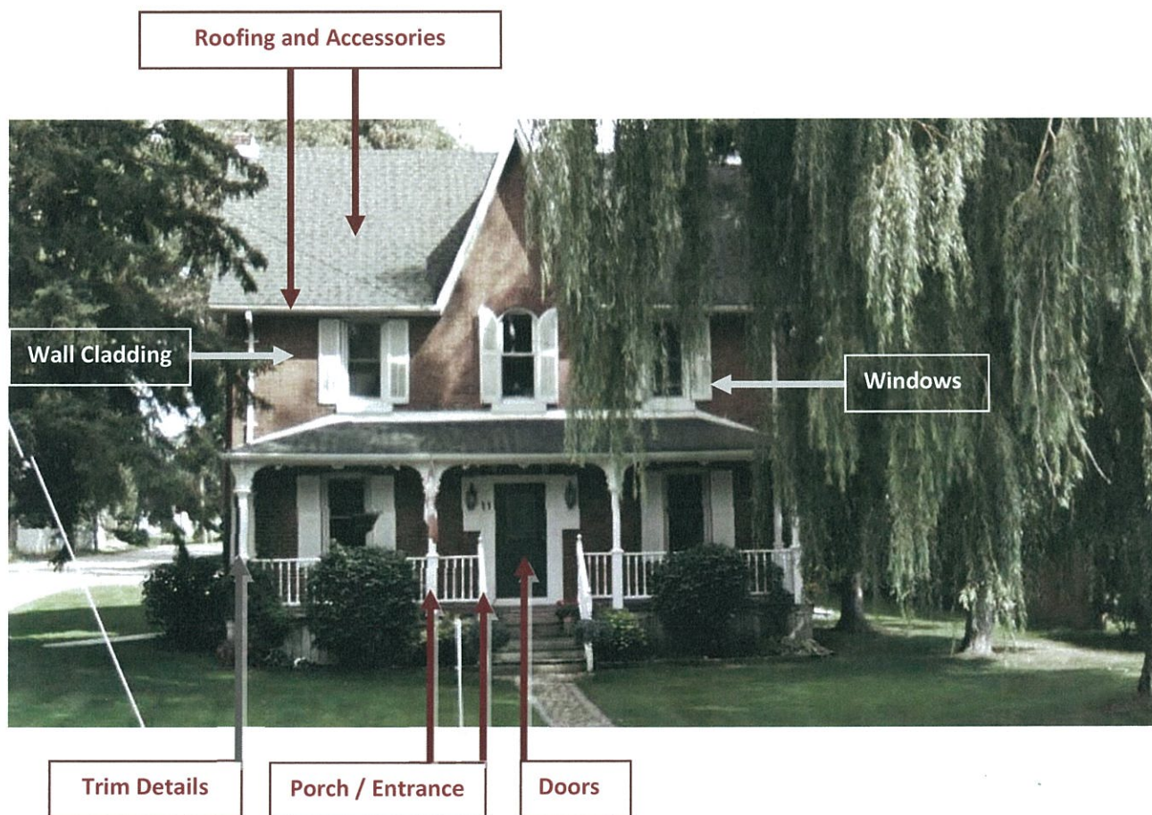
CAMPBELL-BUCHANAN HOUSE 11 King Street North – Heritage Value: High
