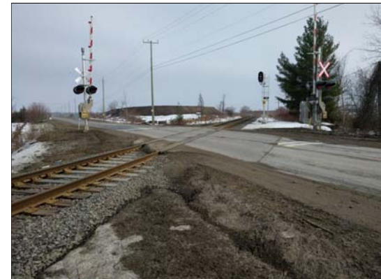
Existing Metrolinx Railway Corridor East of 20 th Sideroad
