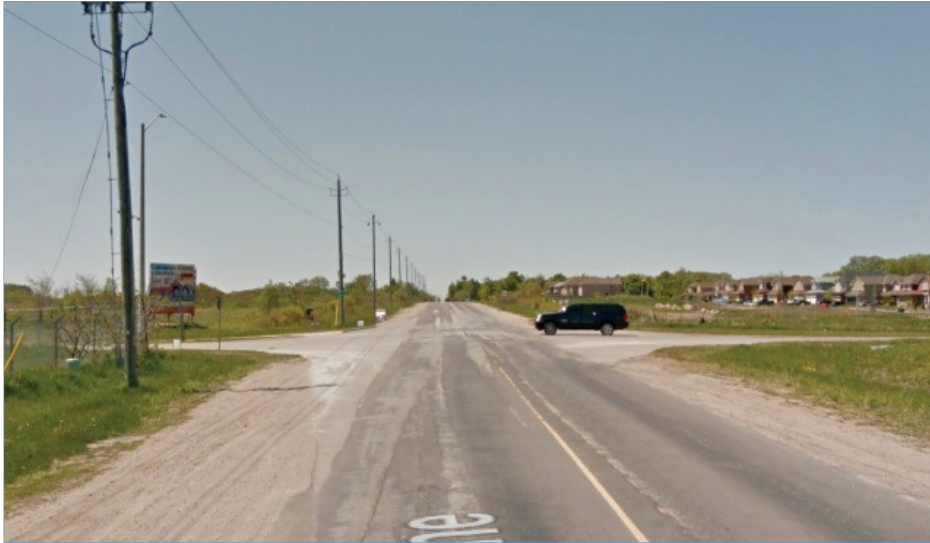
7 TH Line Looking West Towards Webster Blvd.
