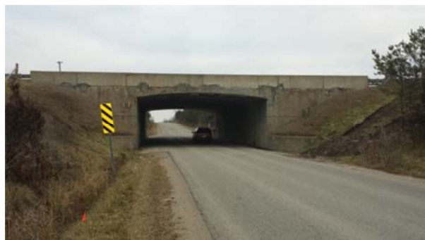
Photo 2: Current Overpass Structure
