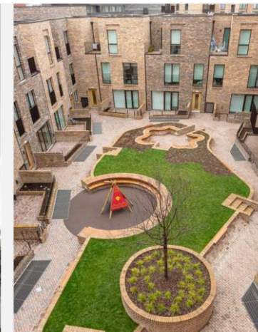
Town houses with communal gardens
